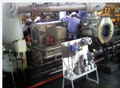
Lubrication system installation
